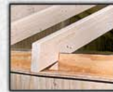
Rafters are notched for extra strength.
