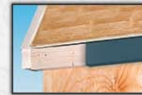
All exposed wood is clad with aluminum.
