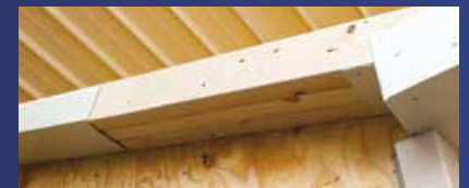
All exposed wood is clad with aluminum or LP Smart Trim (Estate Series)
