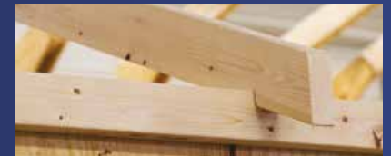
Rafters are notched for extra strength
