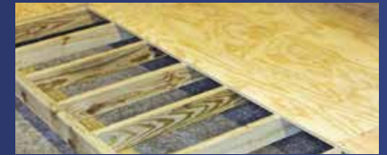
Pressure-treated floor joists
